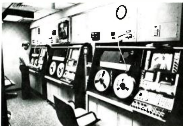
AVR-3s are housed in environmentally controlled room and form the basic VTR capability for ABC's facility.
